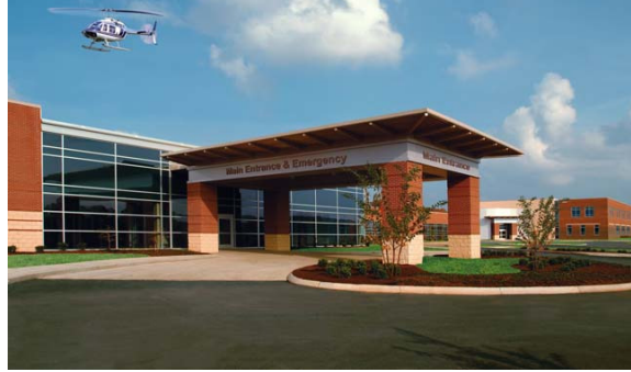
↑ Main Entrance of Medical Center
